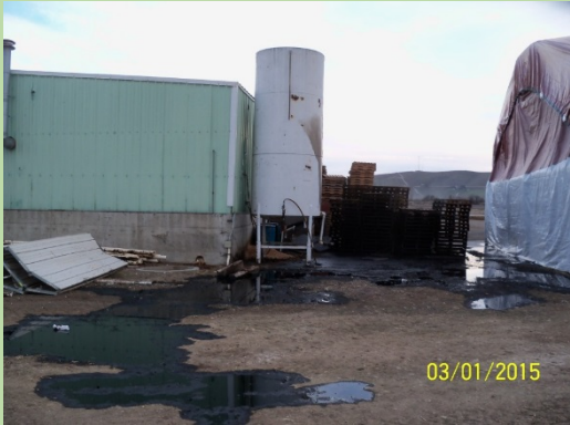
Unmonitored Above Ground Storage Tank fails.
